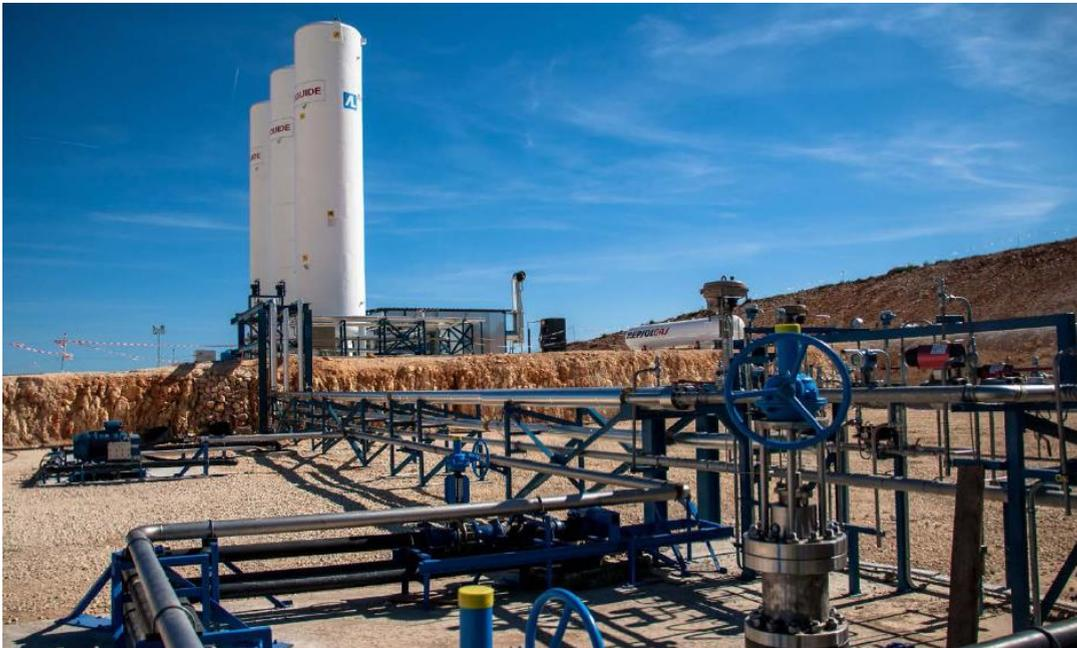
Figure 2: The Hontomin Pilot site: injection infrastructure and CO<sub>2</sub> tanks
