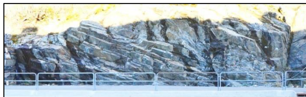
Figure 1. Mannsverk outcrop, 20m-wide, 3-m-high, North is to the left, the outcrop is facing West. The geological scan line was surveyed slightly above the hand rail, from this perspective.
