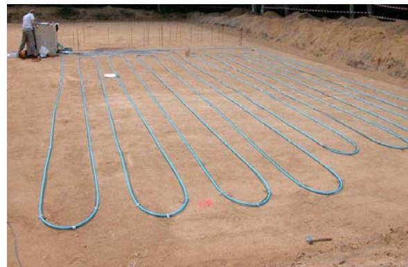
Figure 3: Equipment of one horizontal ground heat exchanger sector by its 2 fluid loops at 1 m depth
